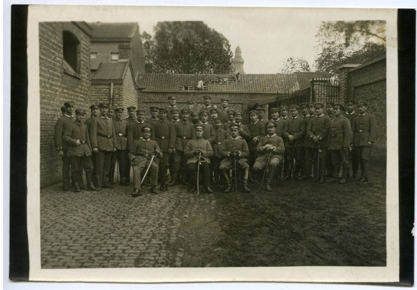
Photo of a group of soldiers with a man repairing a roof in the background (SAG_MA_XII_19_FO_044)
